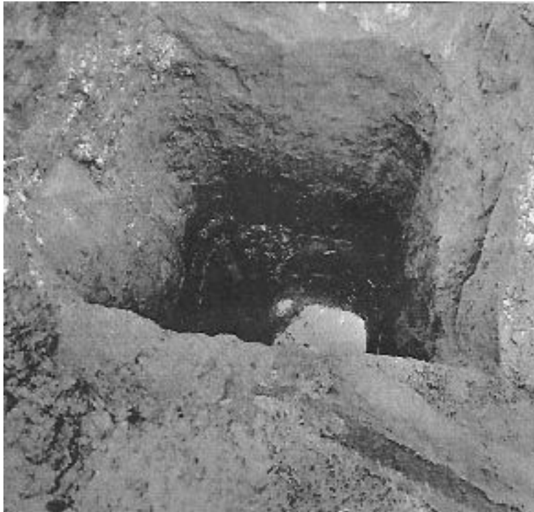
Figure 1: Taken from "Bristol Coal Fields" By John Cornwell. "An unlined mid-18th century shaft found at whitehall in the 1990s. This shaft is sunk through Redcliffe Sandstone which will be about 40 ft thick to work a 5 ft thick coal seam."
